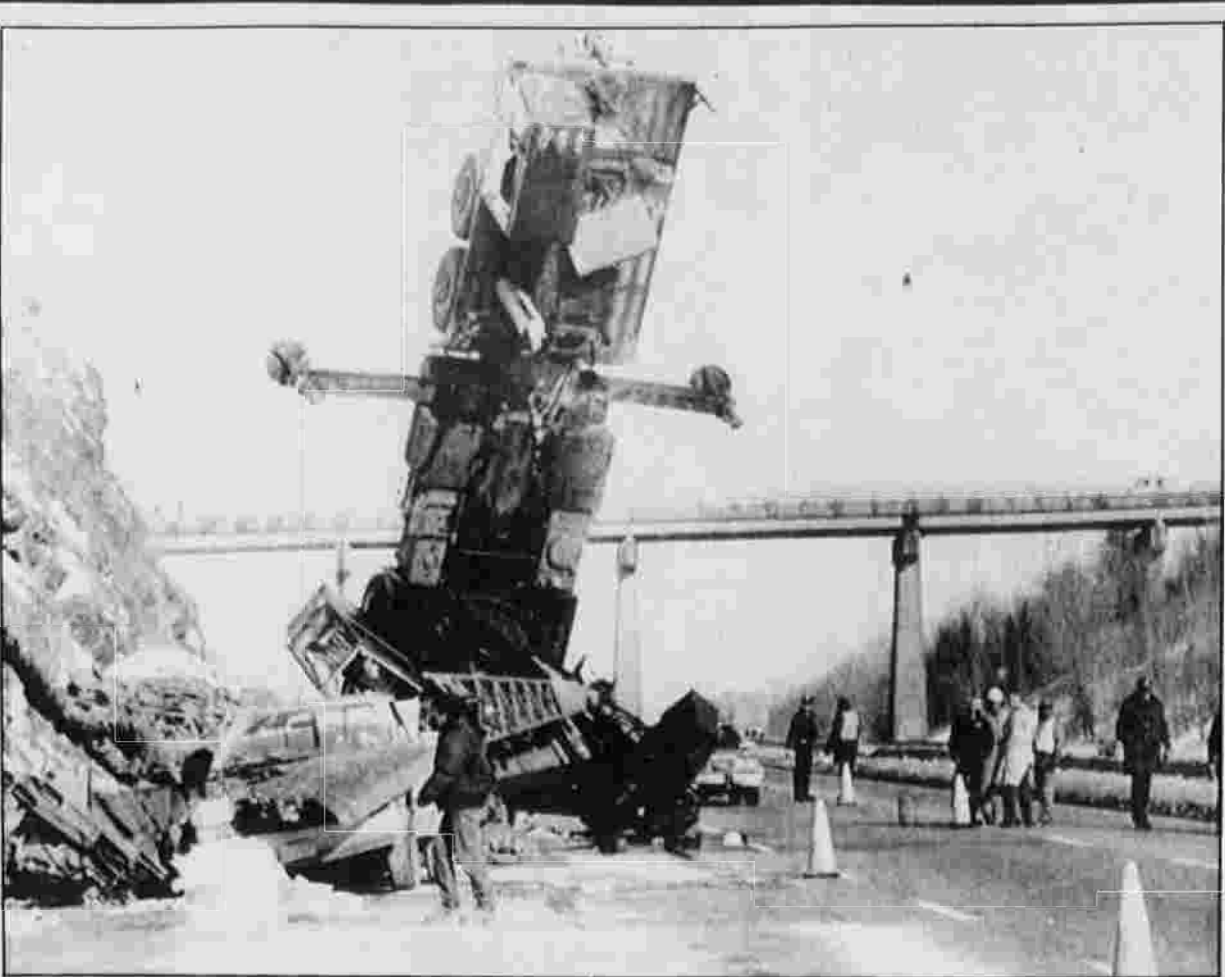
CRANE TOPPLES — The base of a large crane juts into the air in Milbury, Mass., alongside the westbound lane of the Massachusetts Turnpike Tuesday. The accident damaged a pickup truck, but police said there were no injuries.
